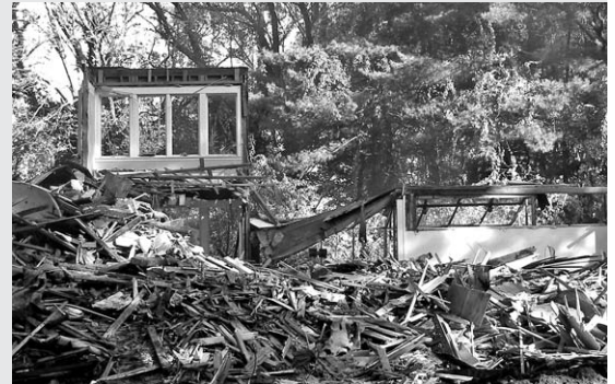
Demolition, Raymond House, Belmont, MA, 2006
