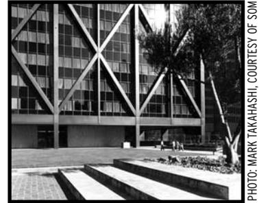
W-SHAPED SEISMIC BRACING AROUND THE BASE WILL ALTER THE PERCEPTION OF THE ALCOA BUILDING FLOATING OVER THE OPEN PLAZA LEVEL.
