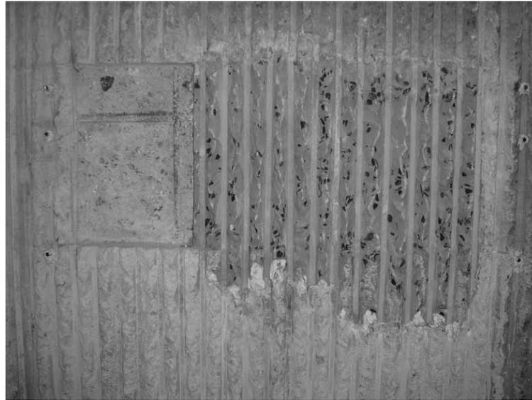
**Testing the making of the vertical 'corduroy' ribs and the adhesion of new concrete to the old, Art & Architecture Building, detail, New Haven, CT.**
